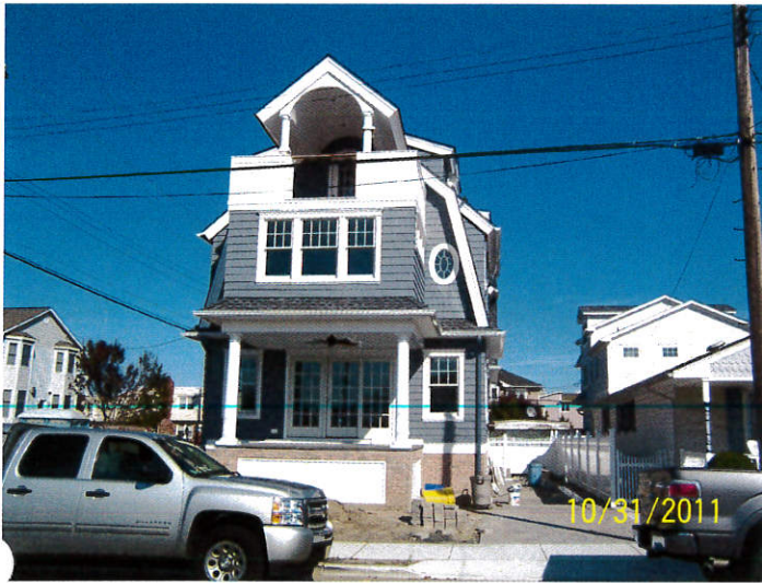
Front View – Date of Photograph: (See Photo Stamp)
